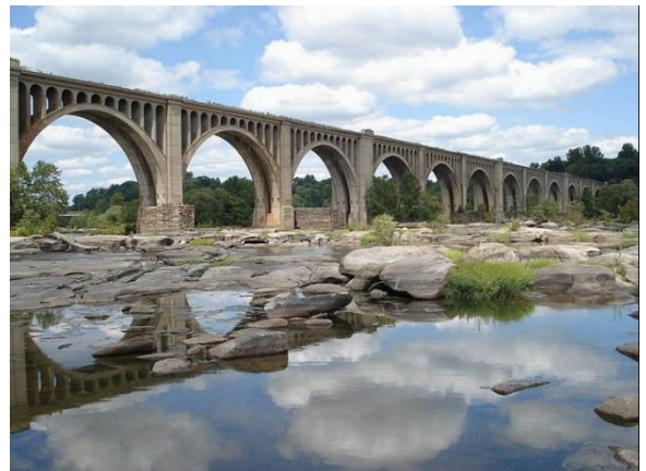
James River Bridge Richmond, Virginia
