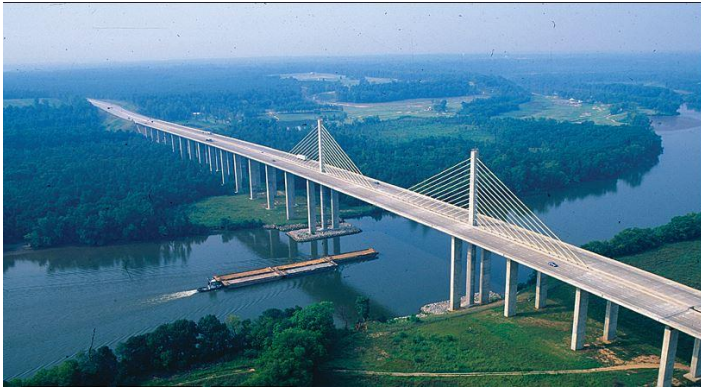
Varina Enon Bridge Henrico, Virginia
